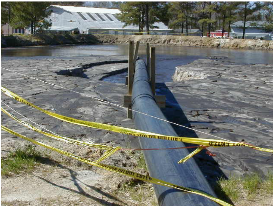
DIKED DISCHARGE AREA WHERE SOCCER FIELD IS NOW LOCATED. ANOTHER SIMILAR DISCHARGE AREA WAS CONSTRUCTED NEAR THE WASTEWATER TREATMENT PLANT FOR DREDGING IN THAT AREA.
