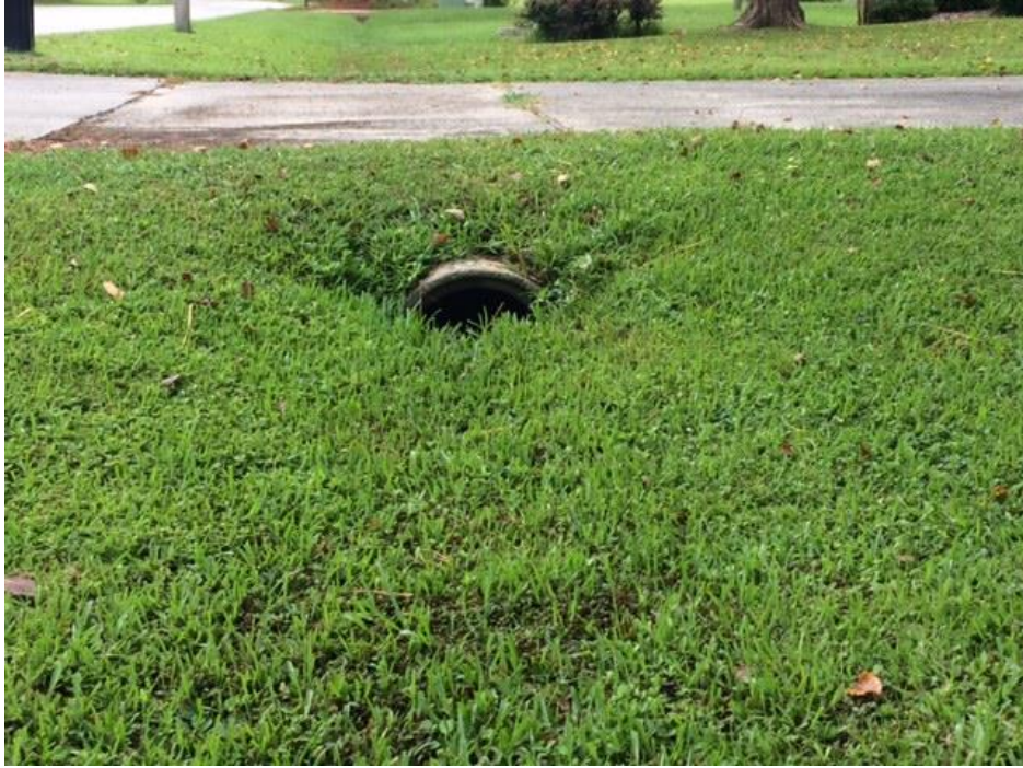
This is an example of a tile that is obstructed by years of accumulation of sedimentation in the ditch.
