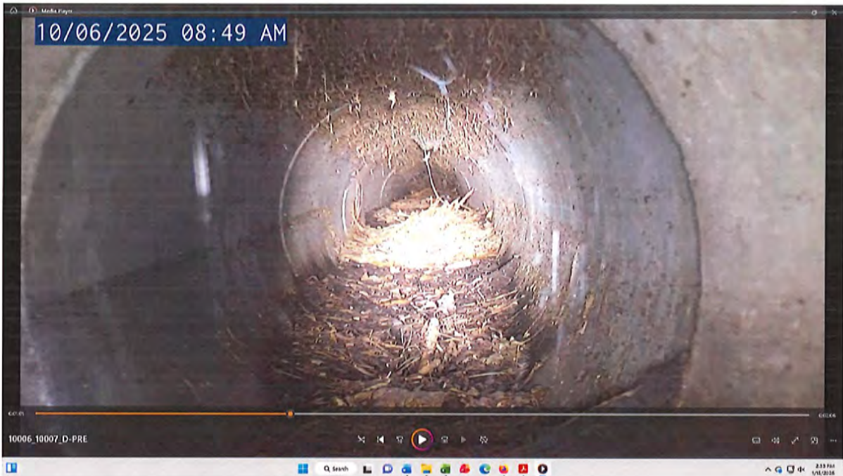
Stormwater Pipe 10006 – 10007: 15 Shoreline Dr.
