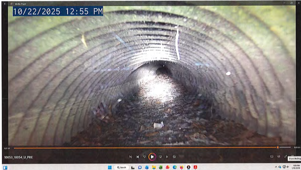
Stormwater Pipe 10053-10054 – 217 Lakemere Dr.
