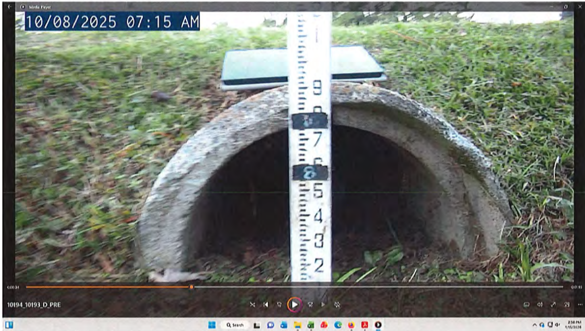
Driveway Culvert 10194-10193: 906 Plantation Dr.
