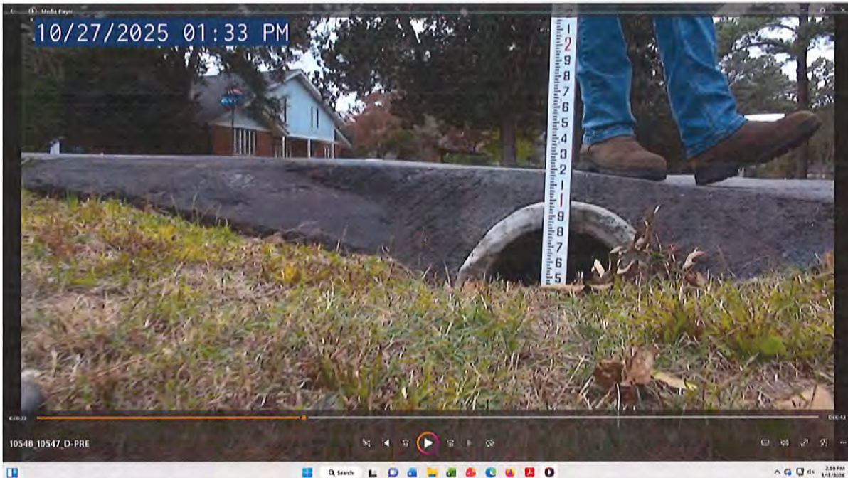
Driveway Culvert 10548-10547: 412 Plantation Drive
