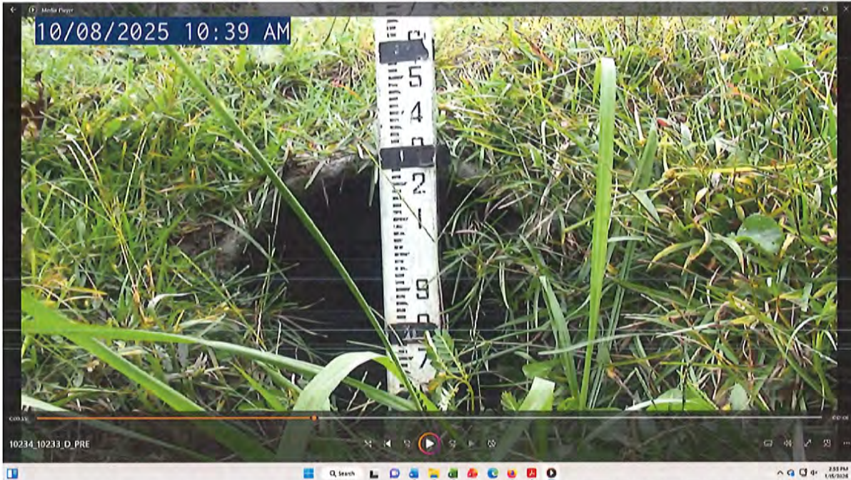
Driveway Culvert 10234-10233: 316 Channel Run Drive
