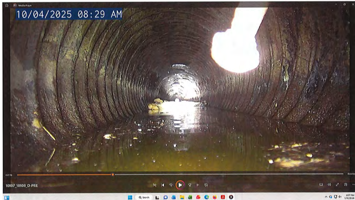
Cross Drain 10107-10108: 200 Bayswater Court (Downstream)
