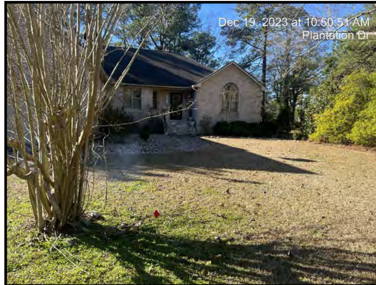
Missing Clean-Out Cap
