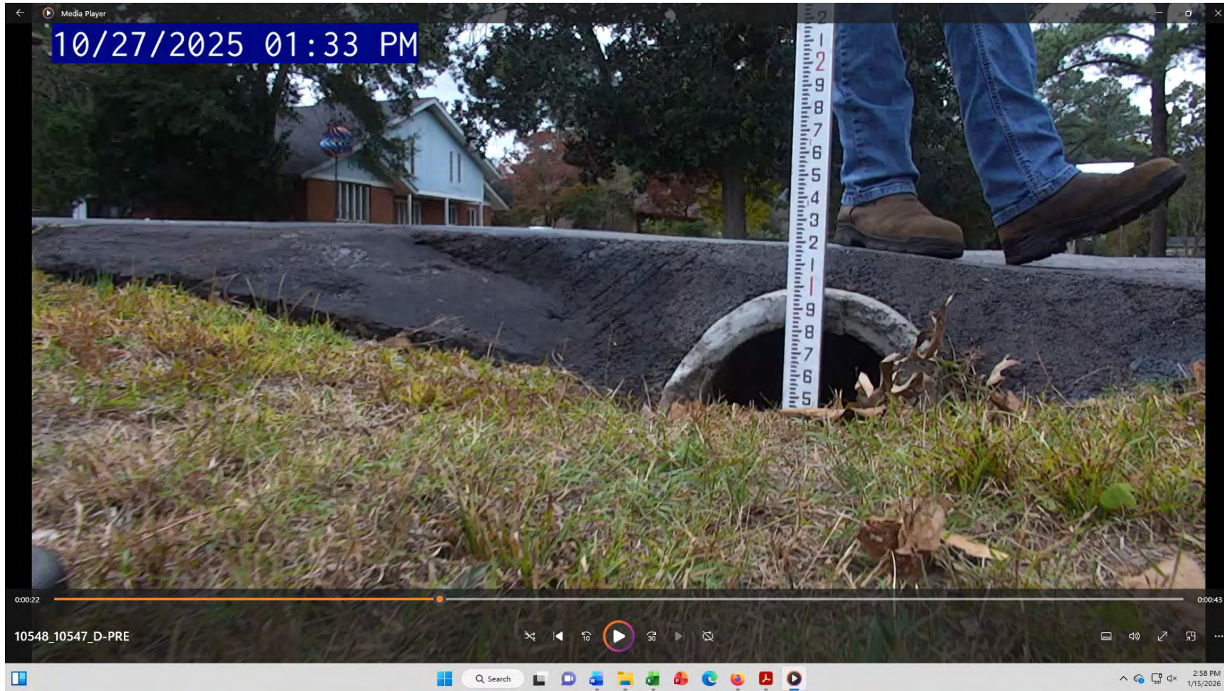
Driveway Culvert 10548 – 10547: 412 Plantation Drive
