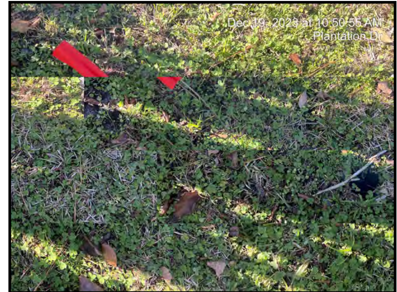
Missing Clean-Out (Inflow Source)
