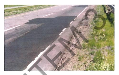
To document pavement areas, measurements were taken with hand tapes and measuring wheels. Where appropriate, area calculations were completed by computer based measurements.
